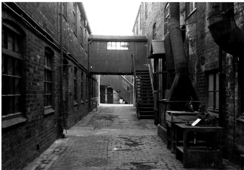
Fig. 11 Middleport after repairs © author
